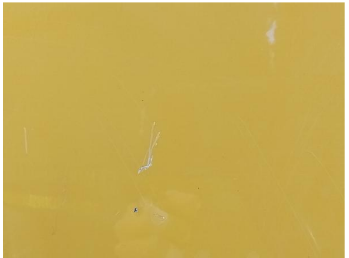
4: Door osf Scratched Over 25mm Thru Paint
